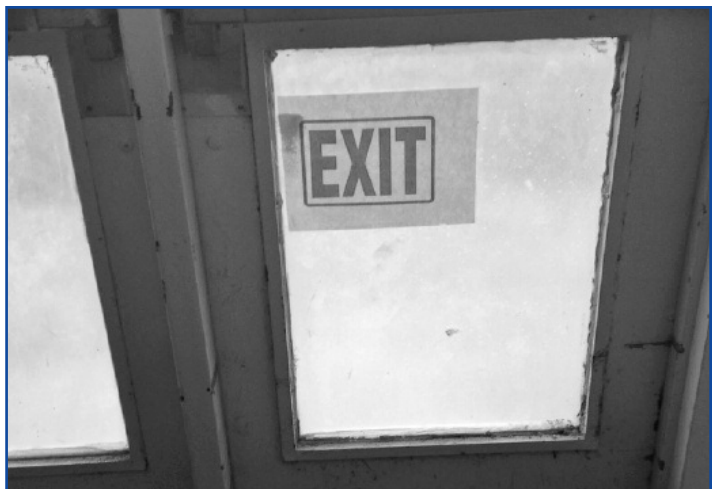
Deteriorated exterior door
