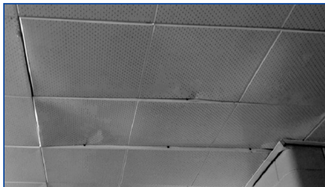
Original corridor ceilings need replacement
